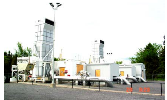
M&I's Exhaust Stack Installation at TransCanada Pipelines site
